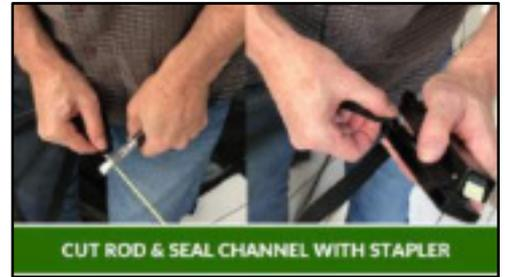
CUT ROD & SEAL CHANNEL WITH STAPLER
