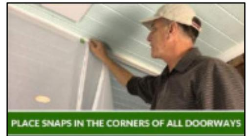
**STEP 3)** Attach the sides of your curtain panels with marine snaps. Begin by sealing all magnetic doorways. Pull panels to edges and decide how much overlap you want on your sealing surfaces. The edge of the panel will extend slightly beyond the edge of your surface.
