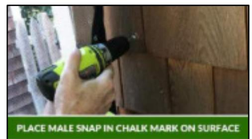
Like magnetic doorways, 5 is a good number of marine snaps to place for applications under 8' tall. Place snaps every 12-18" depending on your wind conditions. Equally space snaps top to bottom. Snap each snap into place from the top and pull down to create vertical tension as you go. This vertical tension makes the webbing lay flat and creates a nice seal against the surface.
